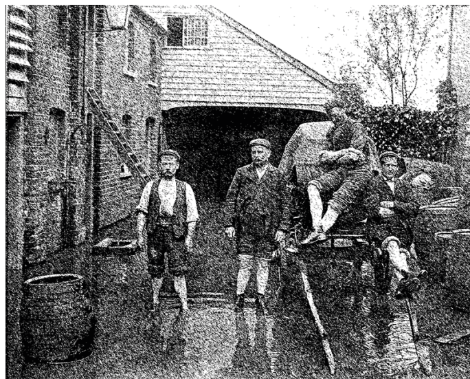
Gardner's Brewery in the flood
