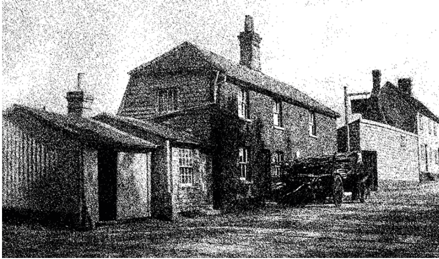
The Tollhouse, Colchester Road
