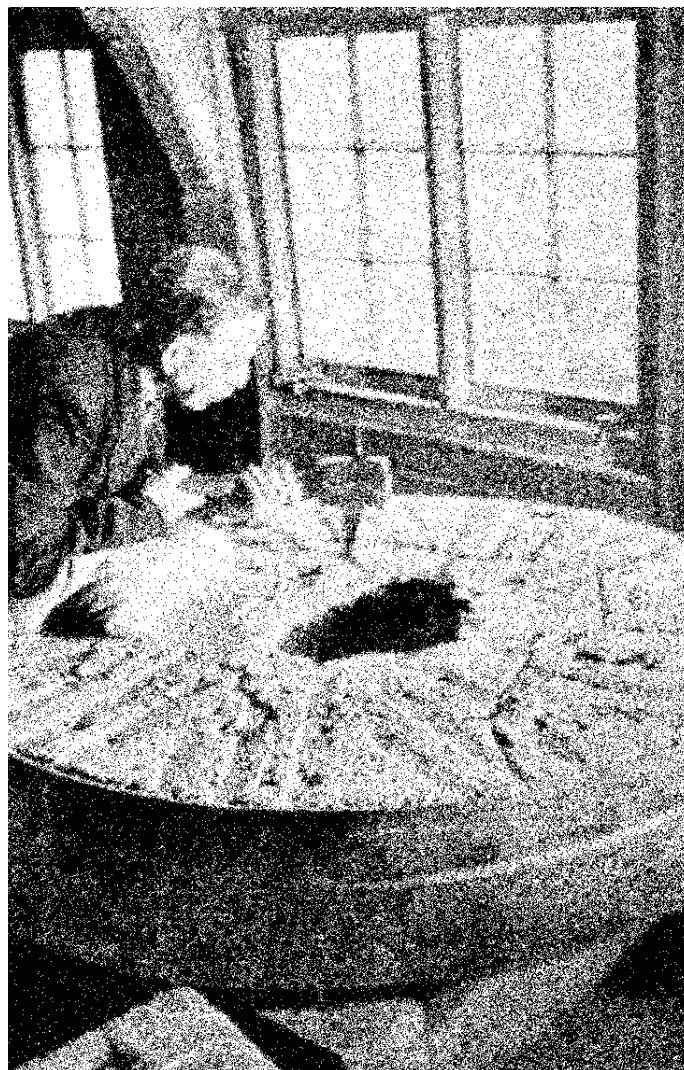
Dressing the millstone, Abbey Mill
